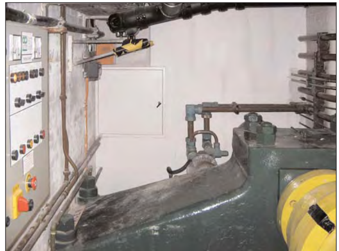
Machine room after airsealing and installation of fire barrier
