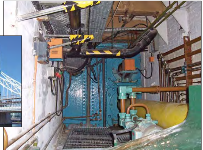
Machine room before airsealing and installation of fire barrier
