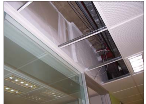
CEILING VOID AFTER
