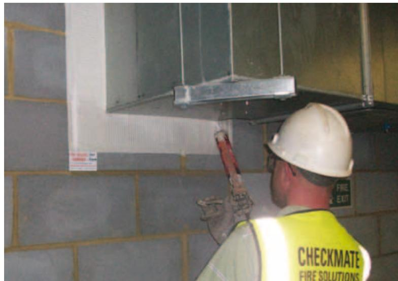
protection, and may not be able to determine issues such as whether or not the linear gap seals to fire walls have been installed to a fire tested detail that will provide the fire rating required. Also, because such items are built into the structure, installation defects at handover stage are often impossible to detect without carrying out destructive tests.
